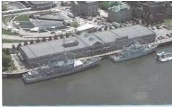
Aerial photos of Pointe-à-Carcy and the NRHQ/CFFS complex
